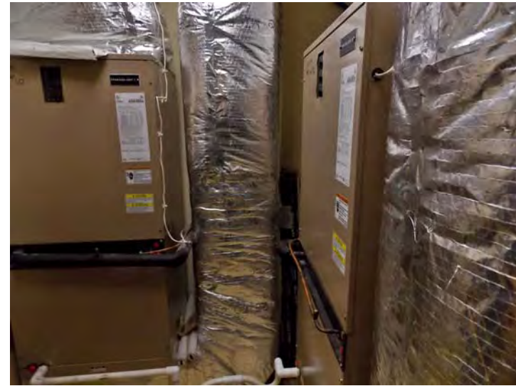
These are the two air handlers (each includes split DX air conditioner coils) that serve the community building.
