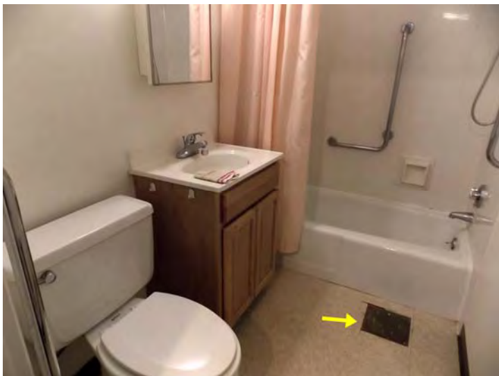
Bathrooms include vanities and vinyl floor covering. Note the missing tile.
