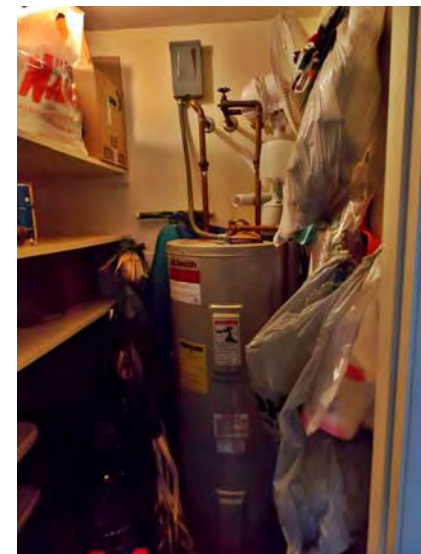
Each apartment has its own electric-heated DHW tank.
