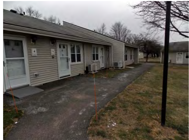
Residential buildings have vinyl-framed windows, direct entry doors, and pitched roofs covered with asphalt shingles.
