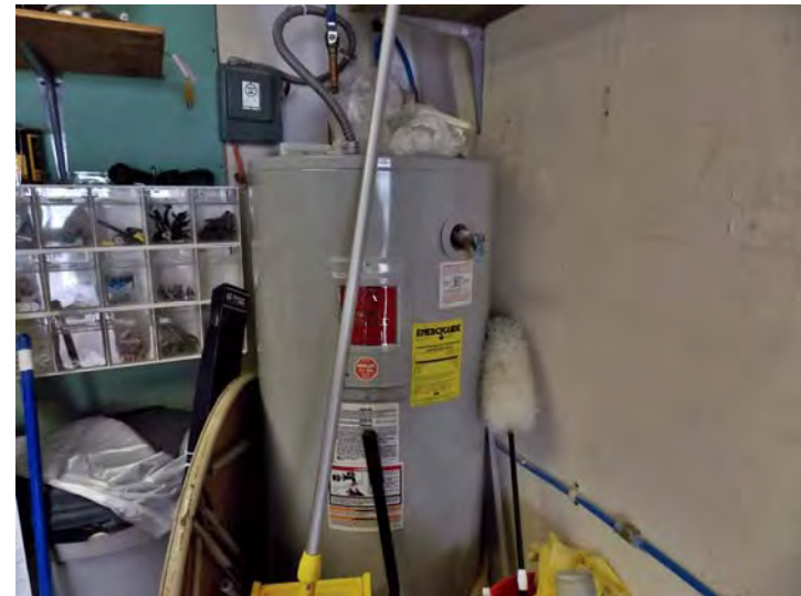
This is the electric-DHW tank that serves the community building (laundry, community kitchen and restrooms).
