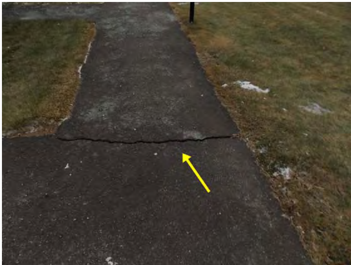
The walkways were recently resurfaced but numerous cracks exist.
