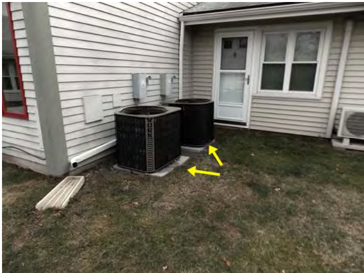
These are air conditioner condensers for a pair of split DX air conditioners that serve the community building.
