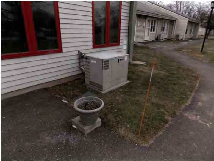
This propane-powered generator provides emergency power to the community building.
