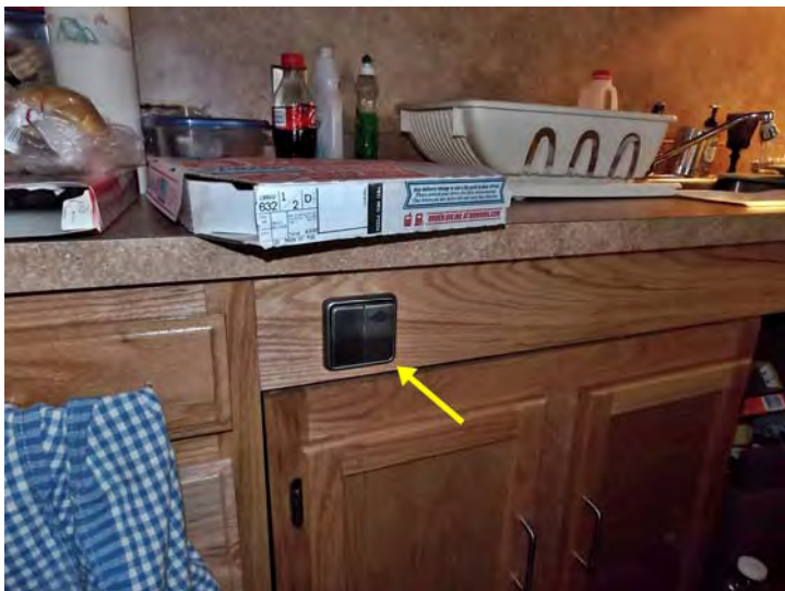
These control buttons are used to automatically adjust the cabinet heights within this accessible unit. Also, the base cabinet is removable.
